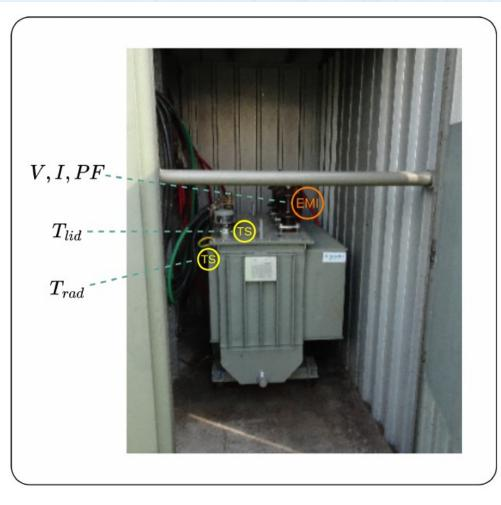
**Figure 5.2:** Suggested final setup for the transformers, with temperature sensor (TS) and electronic measurement instruments (EMI).
