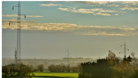
TREFOR Power Grid Living Lab
